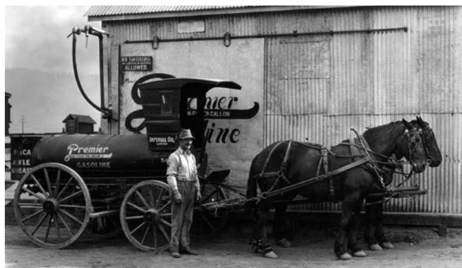
Photo: Kamloops substation with horse-drawn tank wagon, City of Vancouver Search Archives
